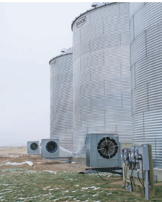
Running aeration fans periodically in the spring will keep stored grain cool.
