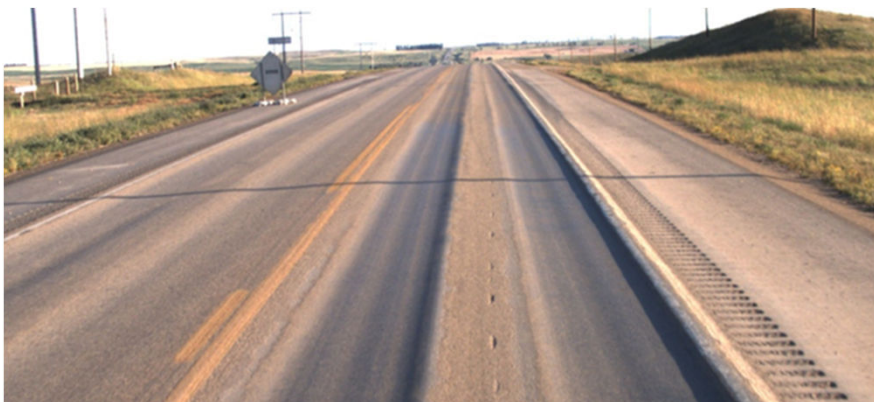
Overweight truckloads cause rutting and other damage to US Highway 85 in western North Dakota during the oil boom.
